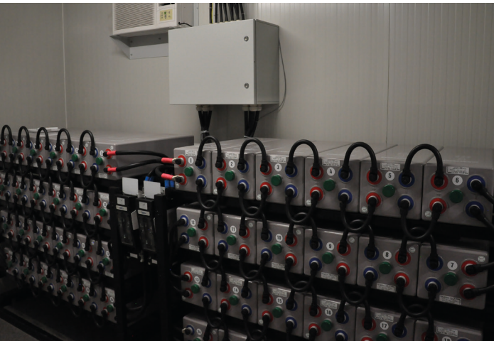
Battery strings housed in the container
