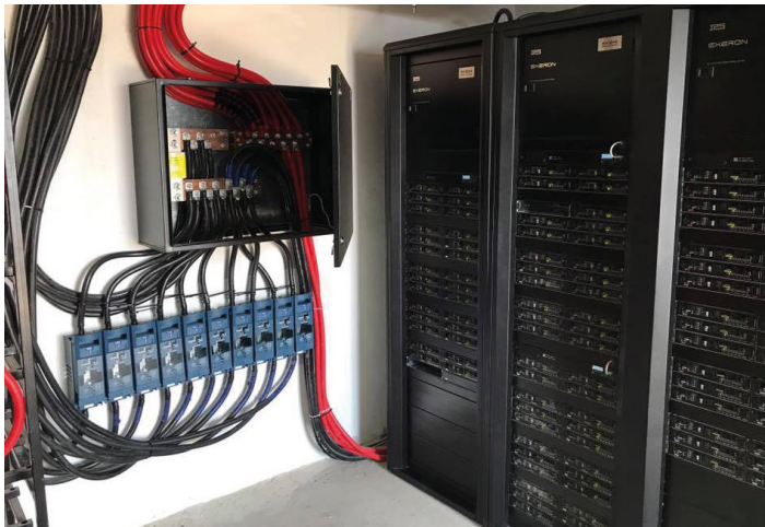
Distribution board and battery fuses
