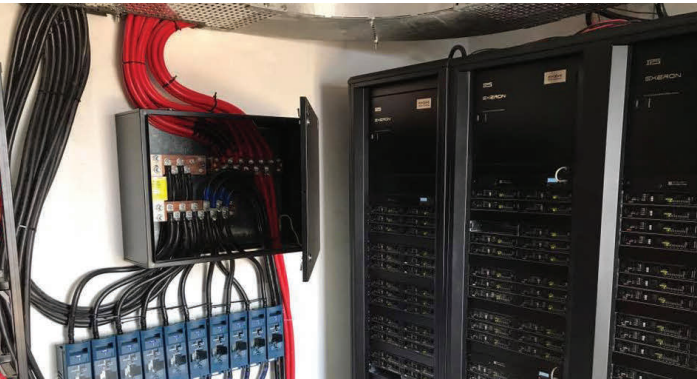
Distribution board and battery fuses
