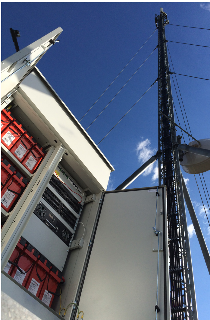
8 kW off-grid power system for TETRA
