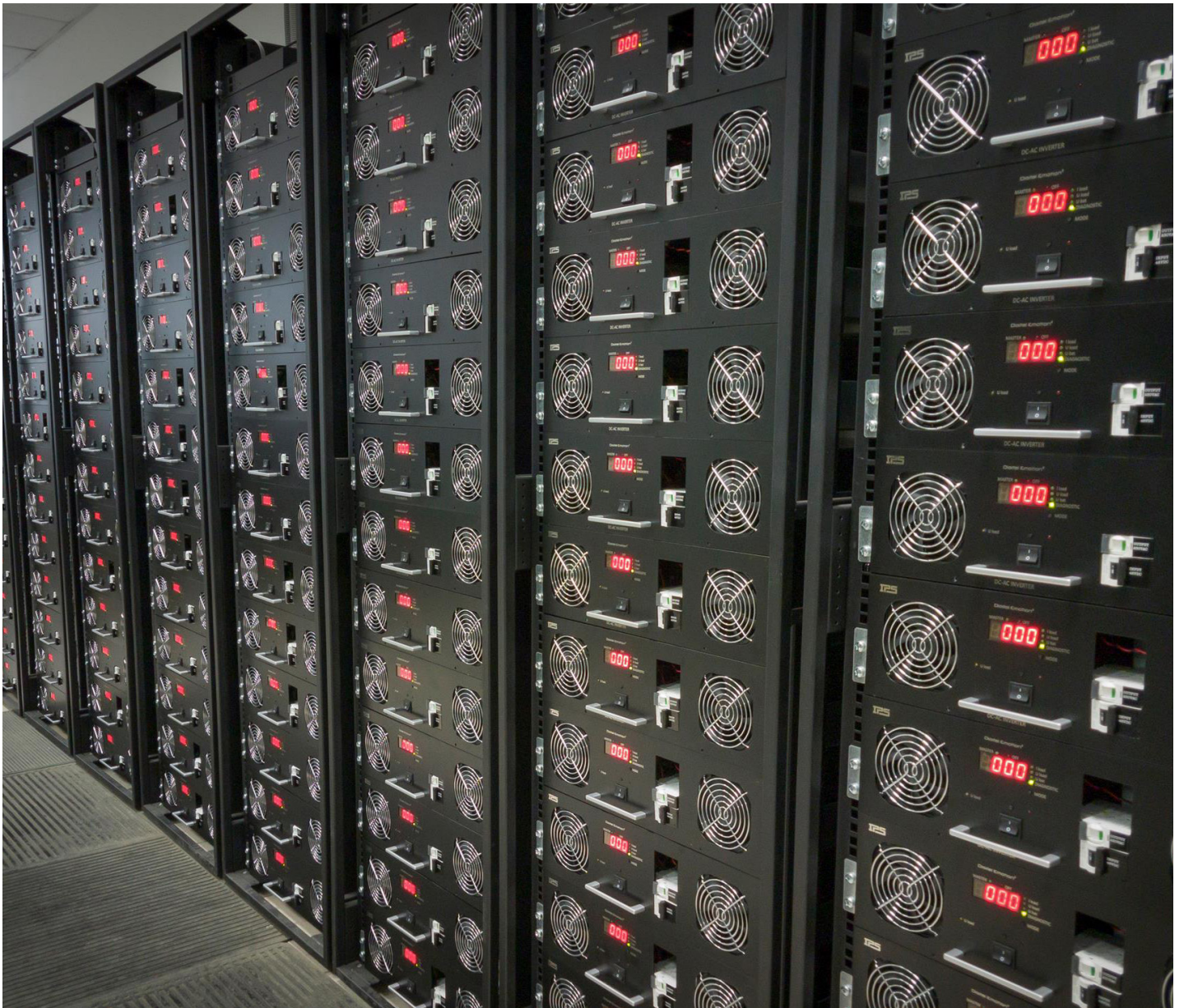
400 kVA Inverter for heavy duty industrial UPS system
